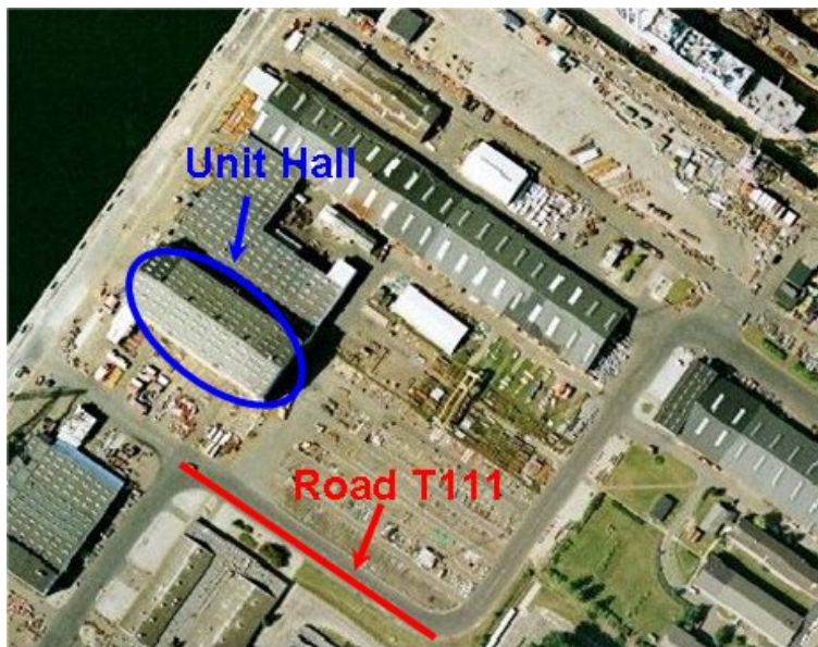
Figure 2.5: Aerial photo of the unit hall and road T111
