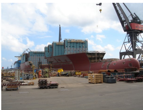
Figure 2.11: Steel sections assembled at the dock
